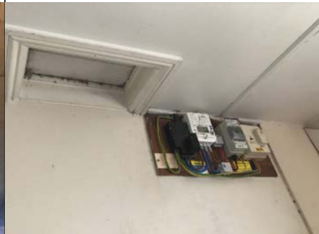
6. View of the mains electrical metering and fuse equipment which is not protected.
