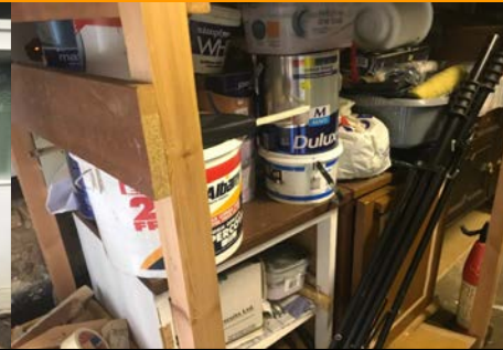
3. There is a high fire loading within the lower ground floor area.
