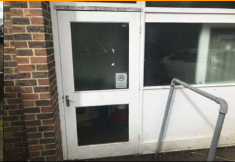
2. Single door exit at front. This will reduce the allowed capacity.
